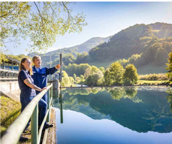
GF operates a hydroelectric power plant on its premises in Traisen (Austria) to generate electricity for its own use.
