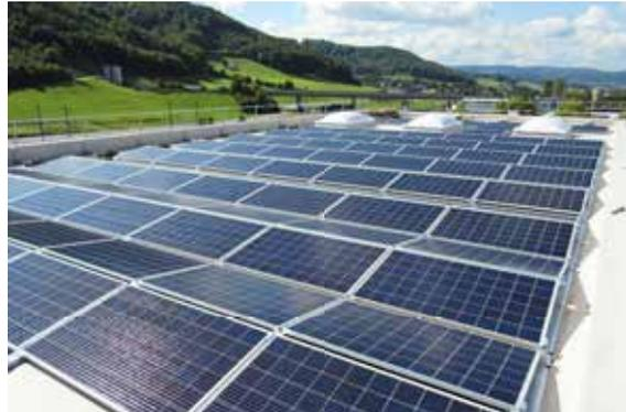
On the roof of the production facility a photovoltaic area of 1'500 m<sup>2</sup> has been installed
